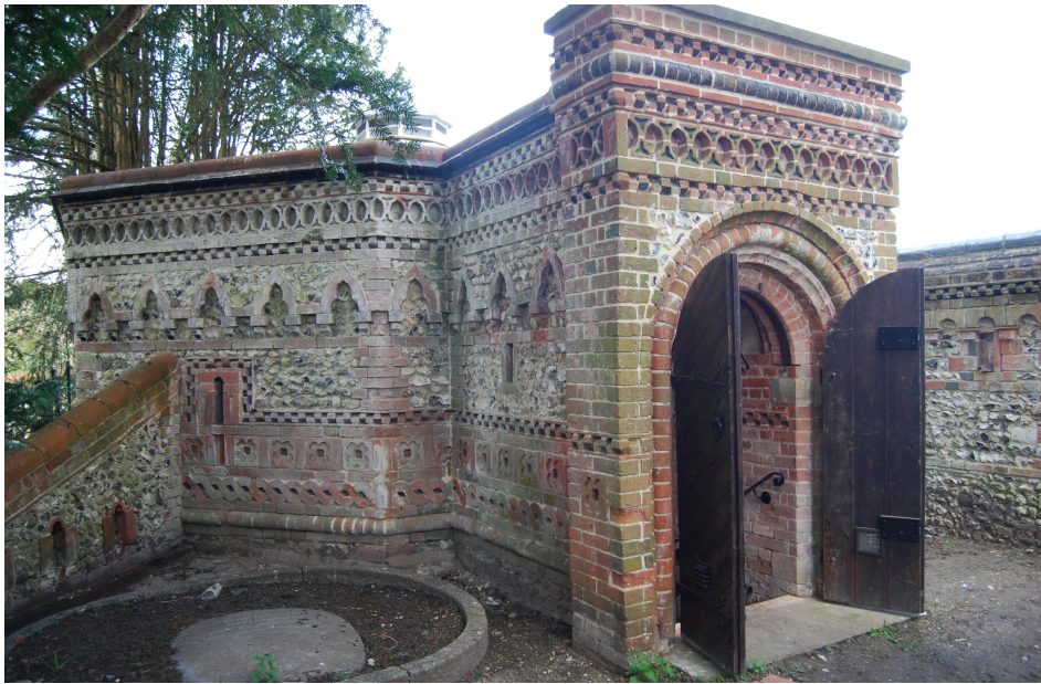
The Lovelace Mausoleum at St Martin's Church, East Horsley was visited as part of the church study day
